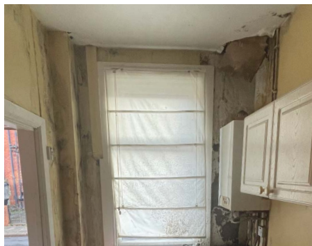
Left - the ceiling has fallen in this kitchen, which is positioned below the bathroom. This suggests a leaking pipe.
