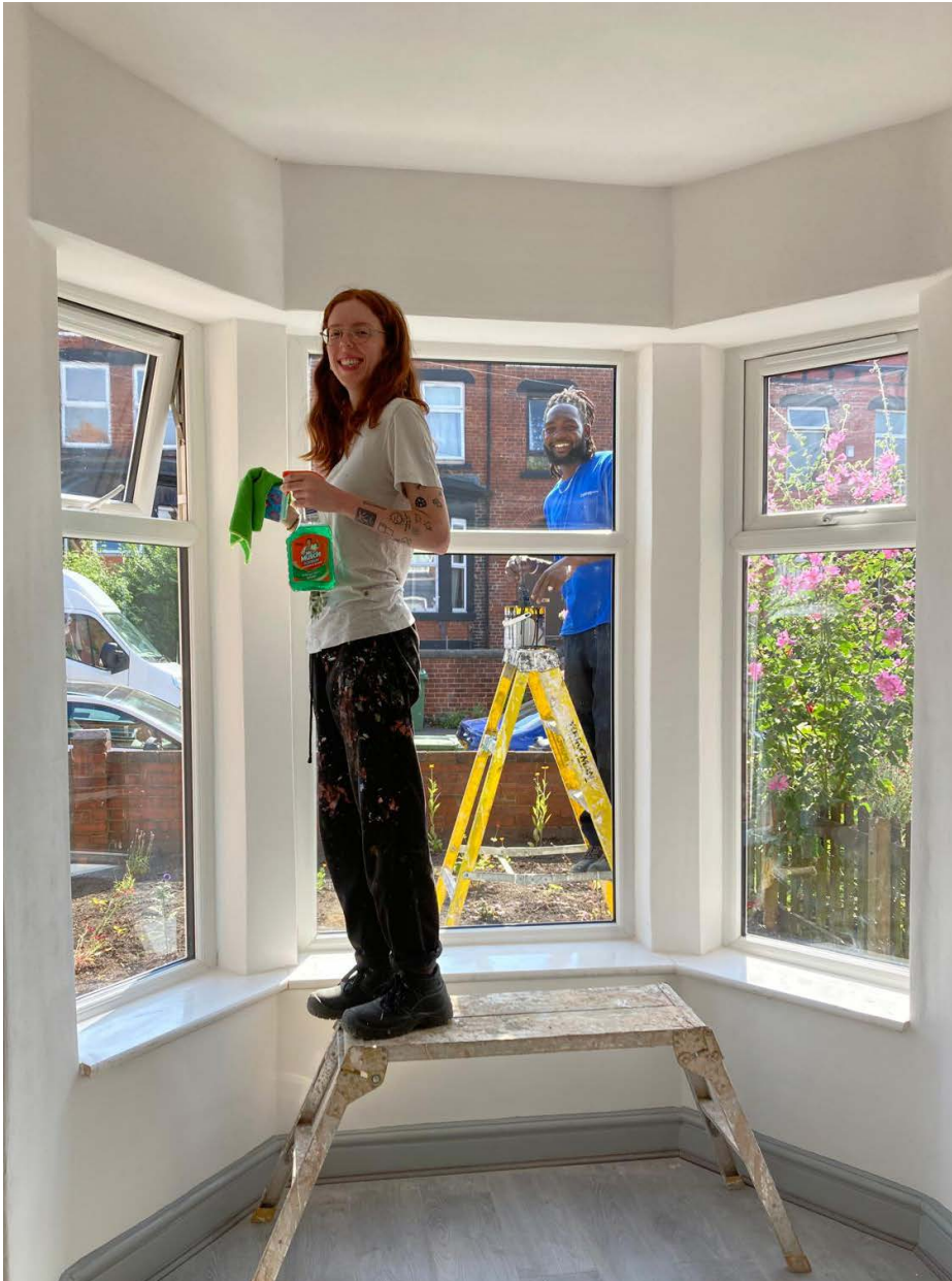
Volunteers finishing up a bay window that has been insulated, lime plastered and painted with vapour-open paint.
