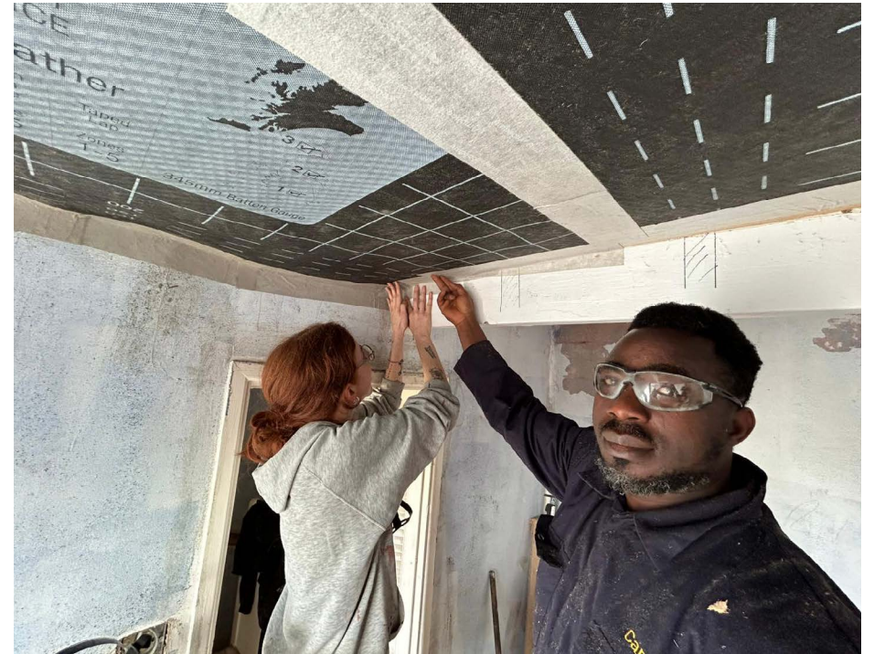
Canopy volunteers fitting and taping an air tight membrane in a dormer roof.
