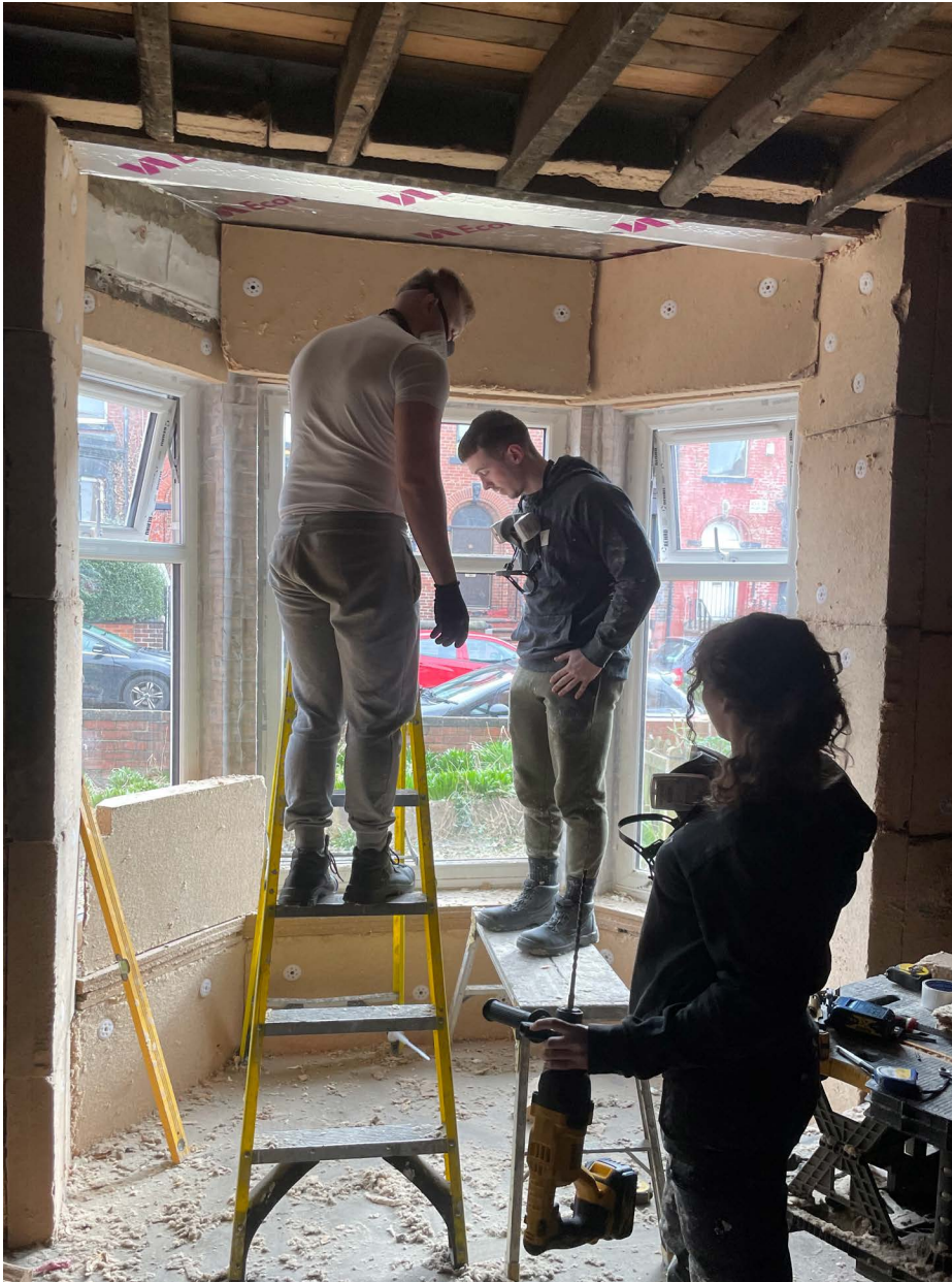
Site workers and volunteers fixing the woodfibre insulation to the interior walls of a bay window.
