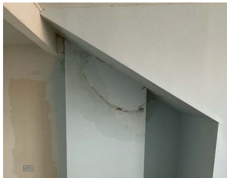
Left - water ingress on chimney breast suggests missing flashing where the stack meets the roof tiles.
